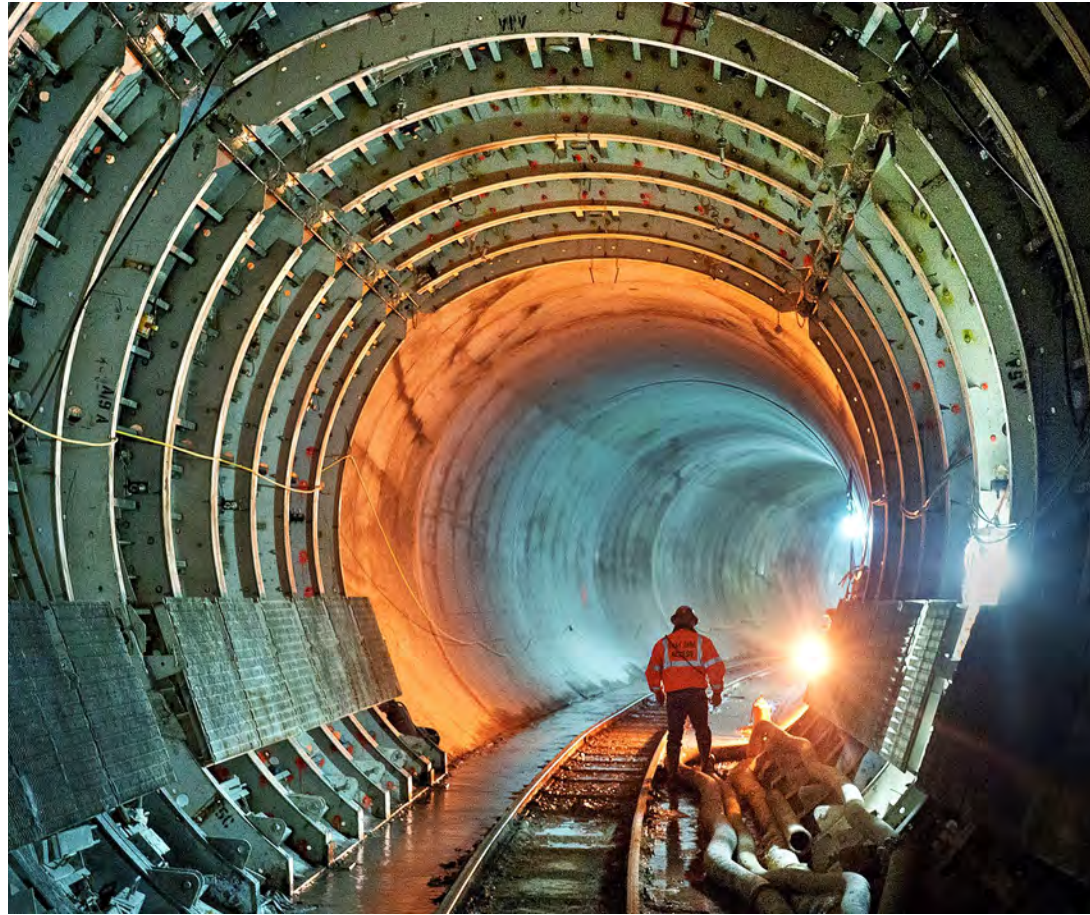
MTA East Side Access, New York, NY
