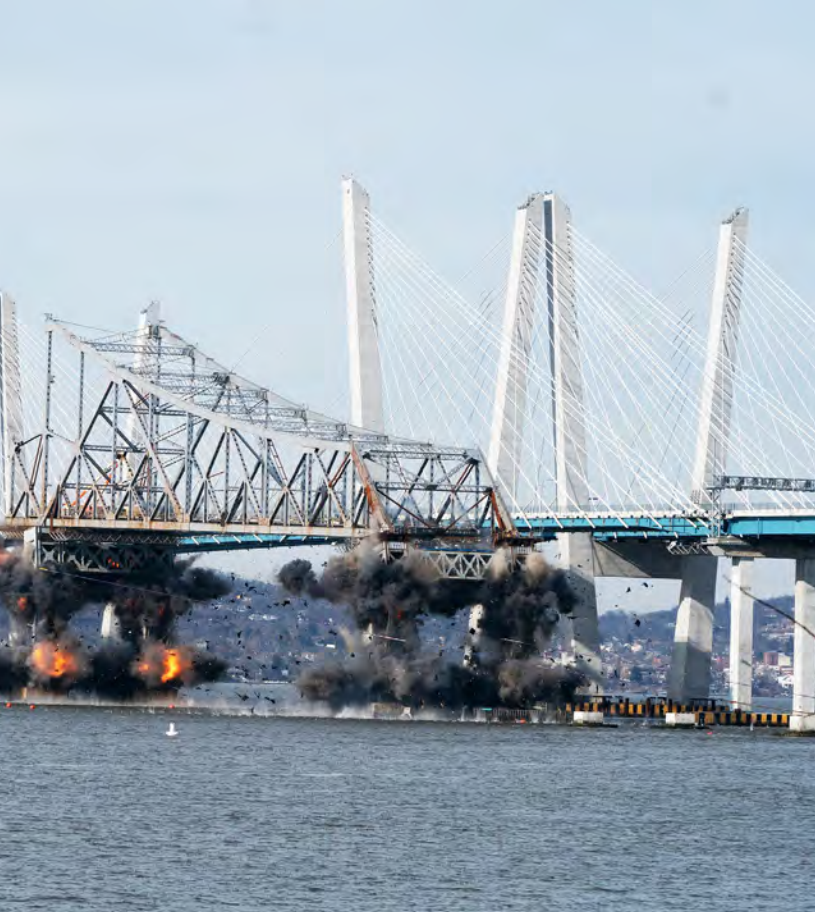
Demolition of Old Tappan Zee Bridge, Rockland/Westchester Counties, NY
