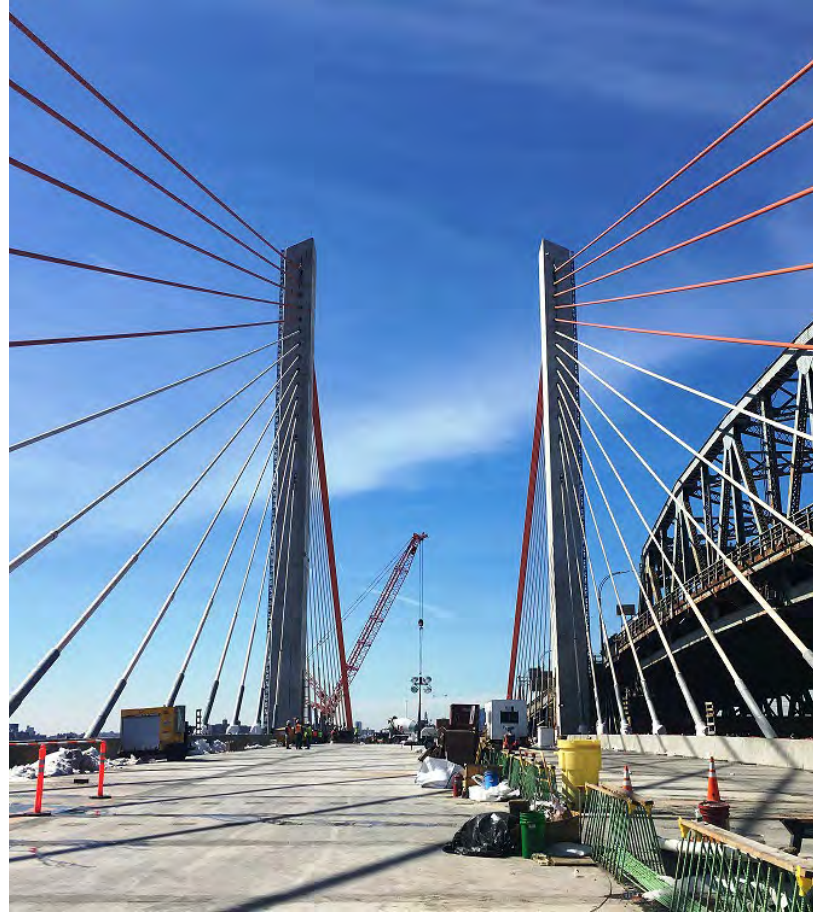
Kosciuszko Bridge over Newtown Creek, Brooklyn, NY
