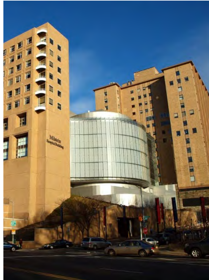
Milstein Hospital Building at New York-Presbyterian/ Columbia University Medical Center, New York, NY
