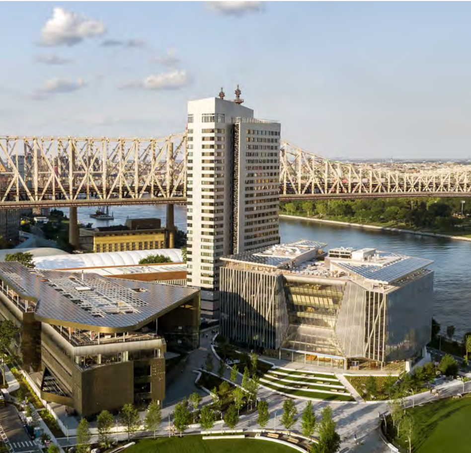
Solar Rooftop Installation at Cornell Tech Campus, Roosevelt Island, NY
