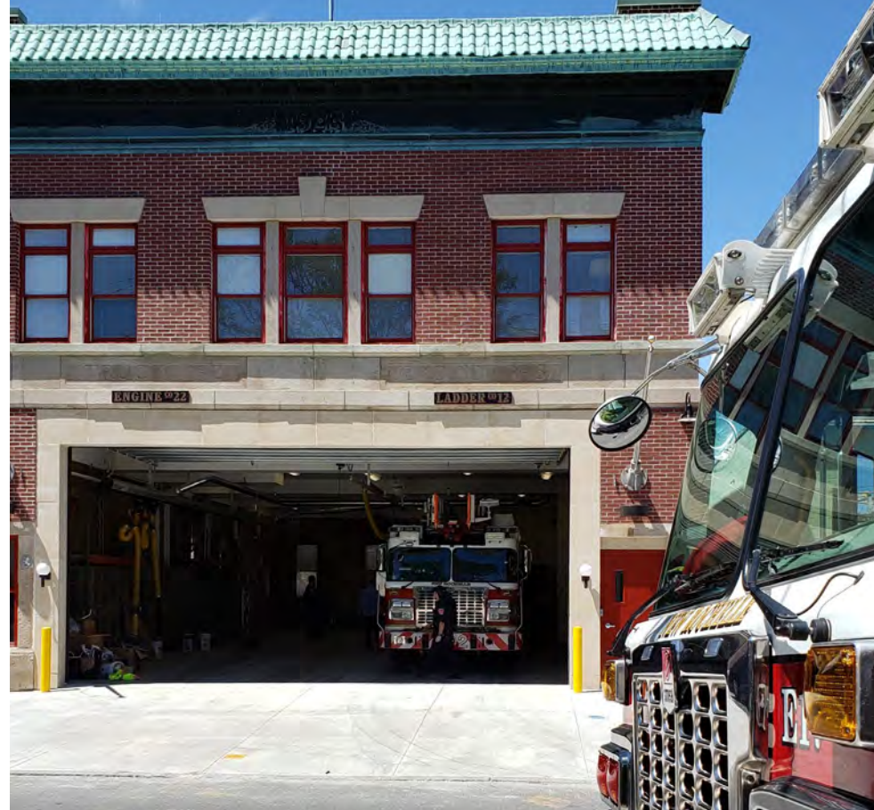
Renovations to Fire House No. 2, City of New Rochelle, NY
