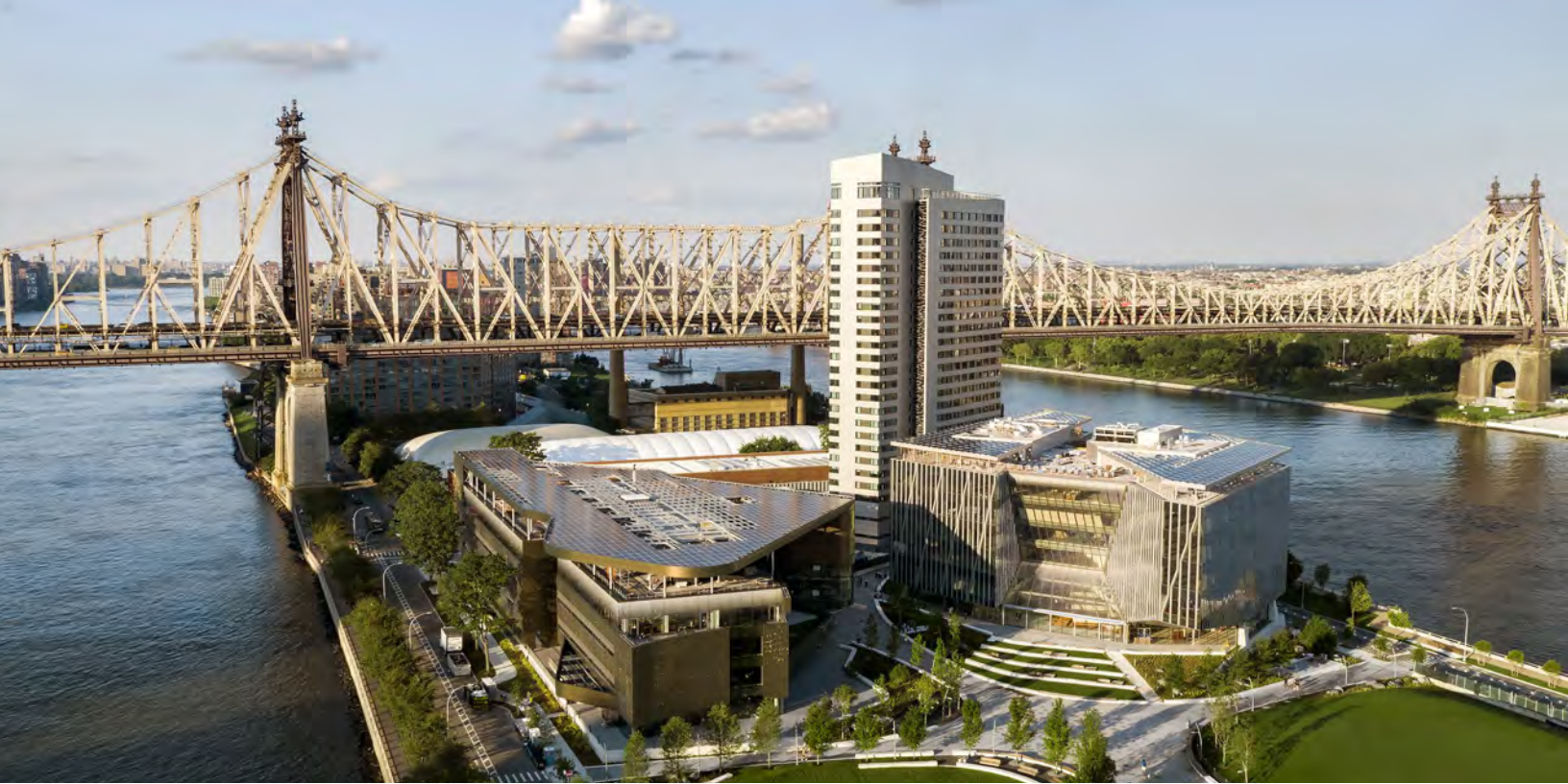
Cornell Tech Roosevelt Island Solar Installation, NYC ACEC NY 2019 Engineering Excellence Platinum Award Winner
