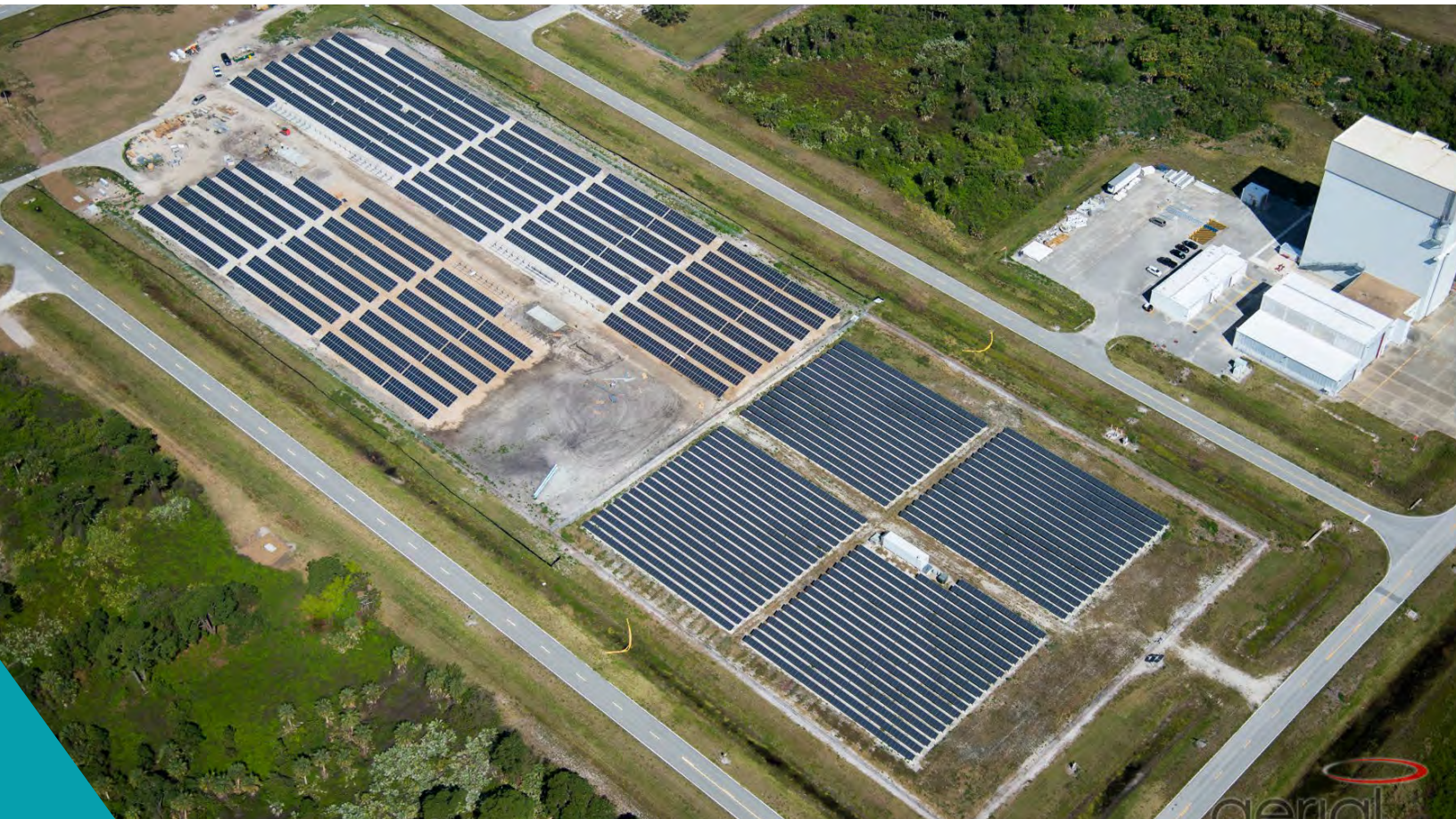
NASA Central Campus Solar Plant Addition, Merritt Island, FL
