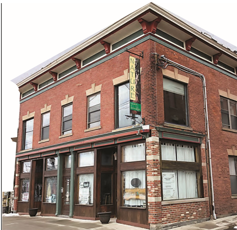
Tectonic is presently providing environmental services to support the County's Division of Planning in connection with federal grant funds they obtained to identify and assess Brownfield sites for reuse and redevelopment in Sullivan County, focusing on the urban centers of Monticello, Liberty and South Fallsburg, NY
